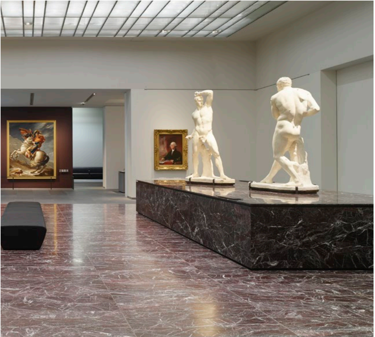
covering: red levanto panel core: calcium sulphate dimensions: special size
